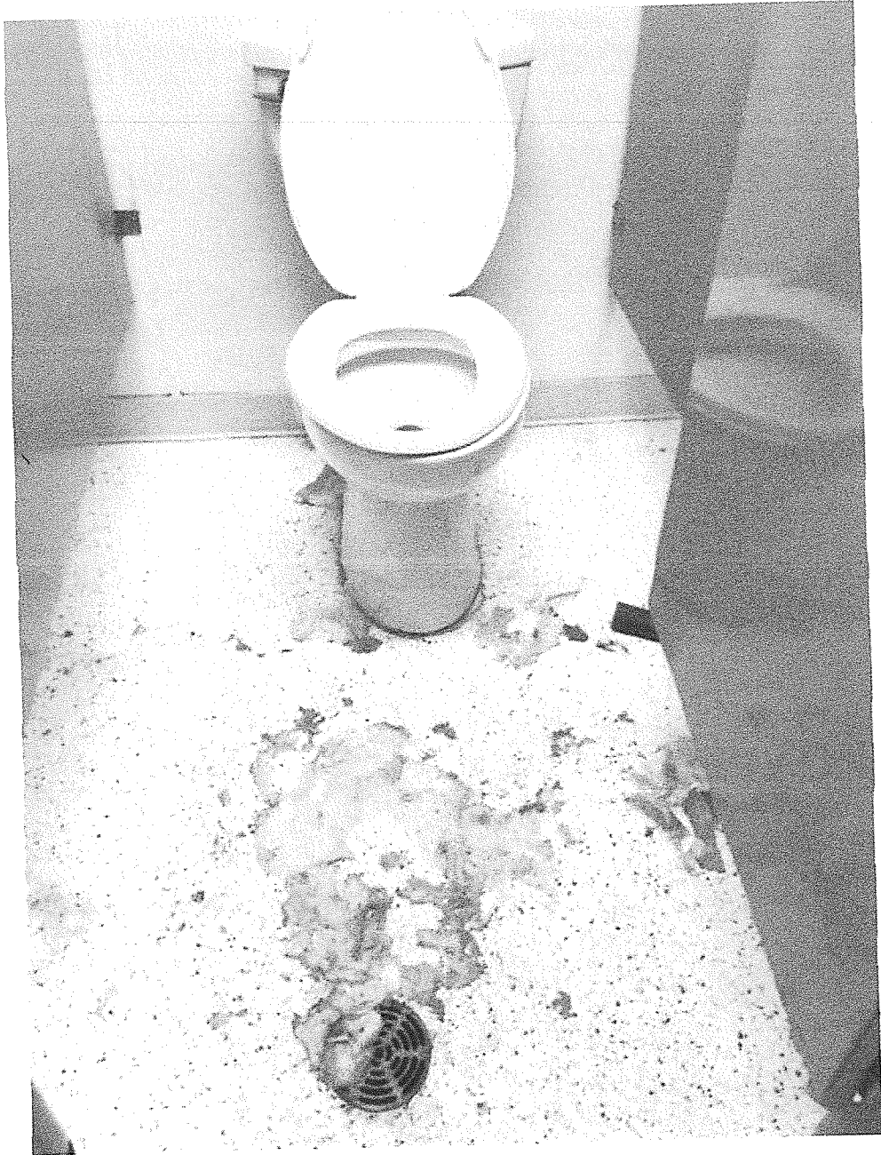
Pavilion ladies restroom 7/4/18
