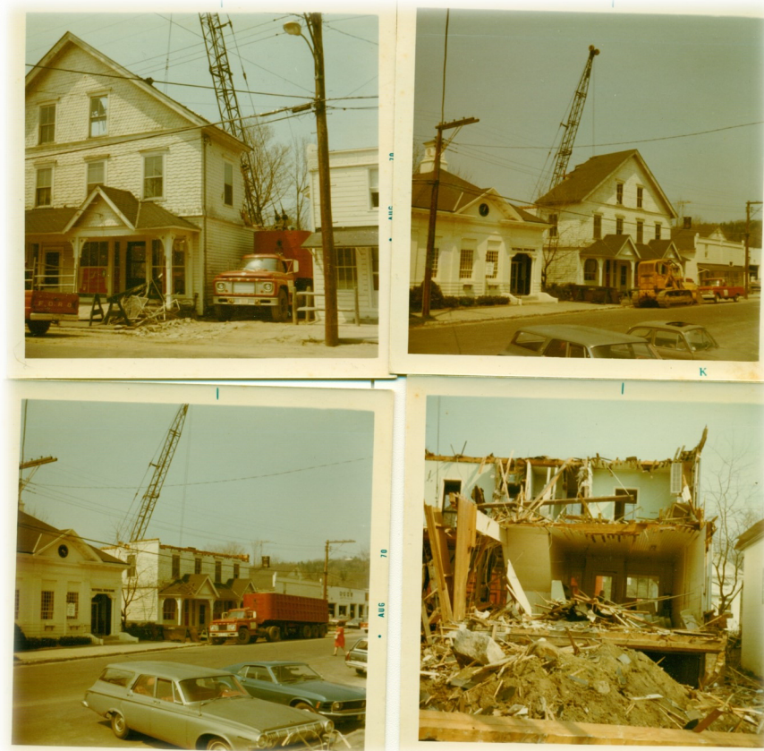
Demolishing Bergenty's Store
