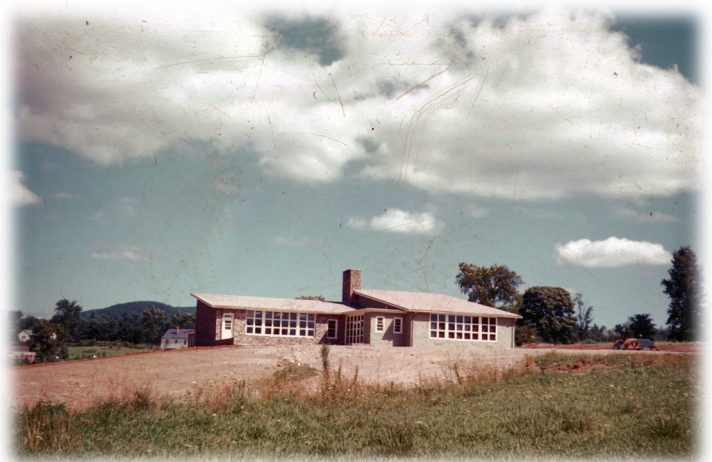
Newly constructed Lee H. Kellogg School
