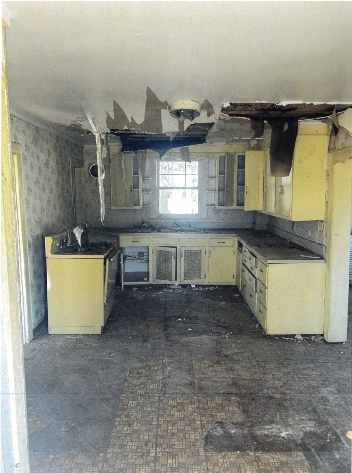
Picture 13: First Floor Kitchen – Ceiling sections are actively collapsing, exposing structural framing and creating an imminent risk of injury. This level of deterioration indicates severe water infiltration and compromised load-bearing integrity.
