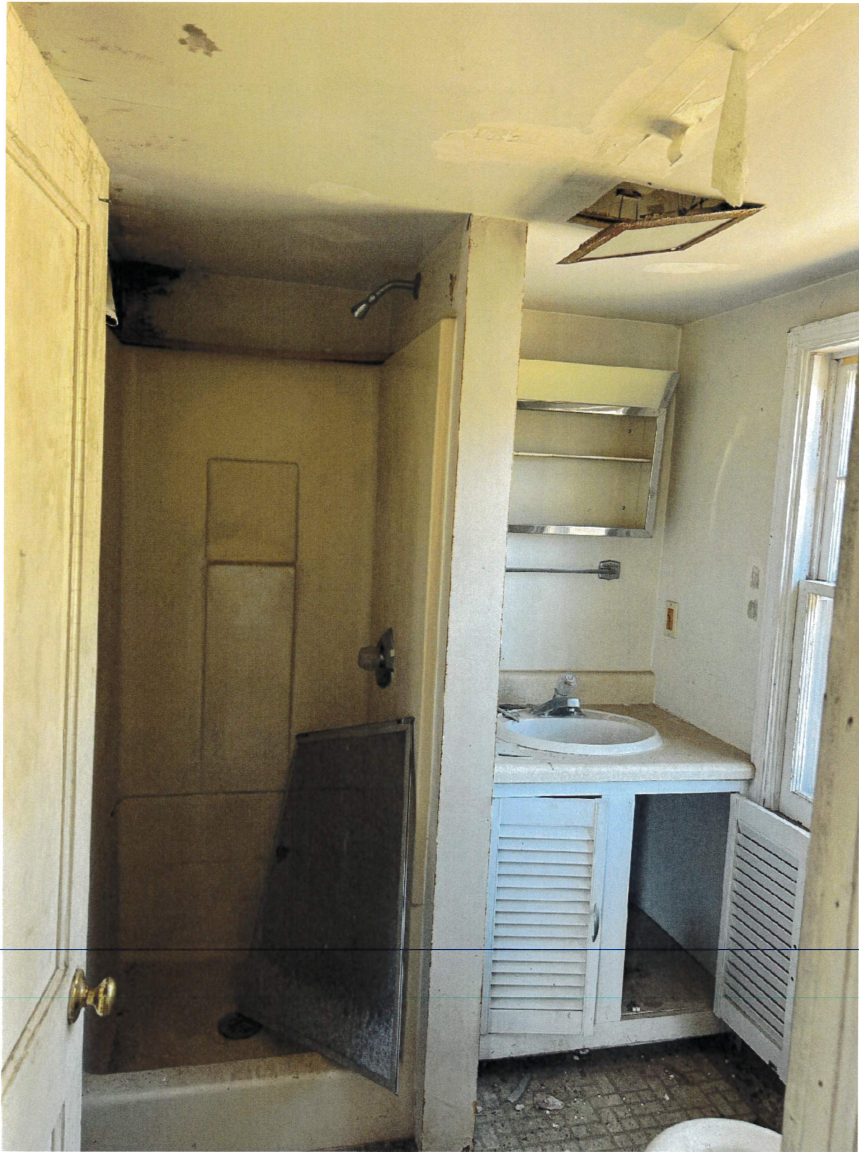
Picture 17: First Floor Bathroom – Damaged and non-functional light fixtures in the bathroom underscore the unsafe electrical system.
