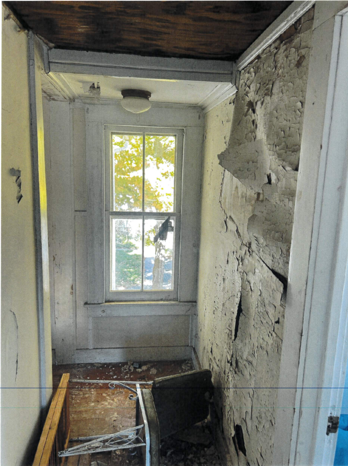
Picture 9: First Floor Hallway – Exterior and interior surfaces show extensive peeling and rotting paint, indicating prolonged moisture exposure and wood decay. This level of deterioration compromises structural integrity and reflects years of neglect.
