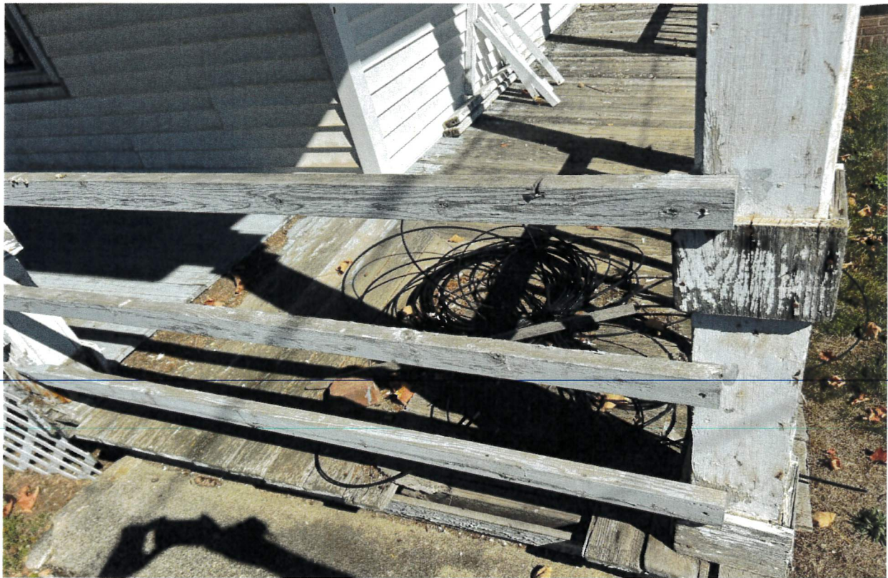
Picture 4 (Bottom Picture): Front Porch - Structural instability and advanced deterioration of support
