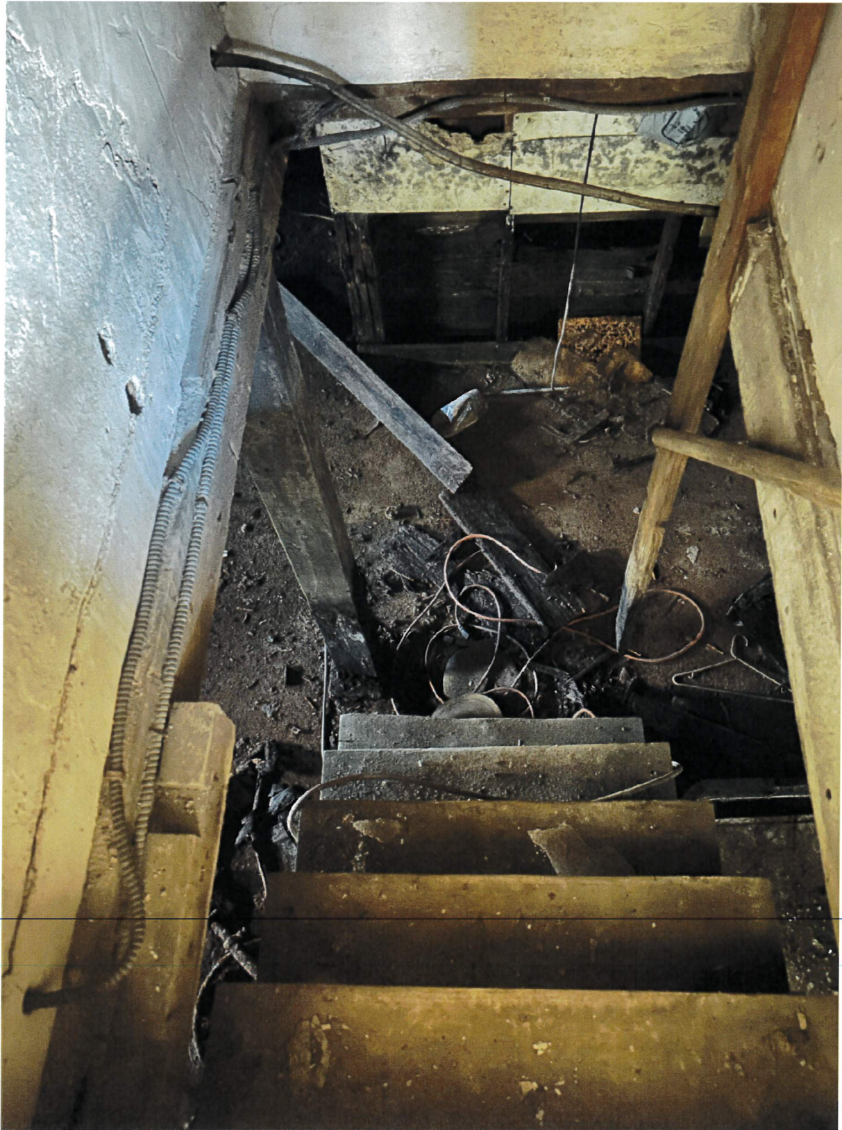
Picture 16: Stairway to Basement – Shows exposed electrical wiring and unsecured plumbing along the descent, creating severe fire and water hazards. Missing steps at the bottom make the staircase unsafe for use.
