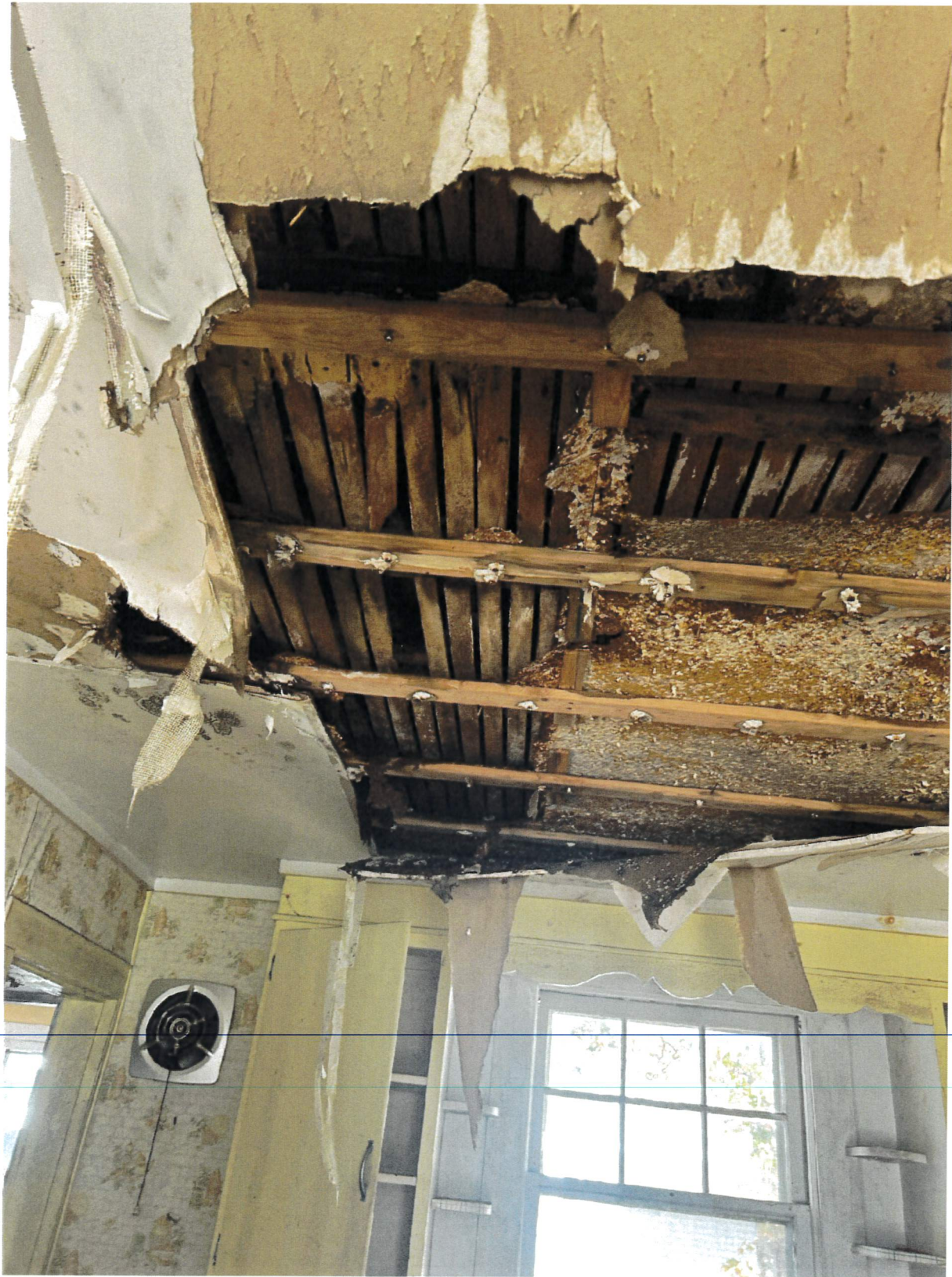
Picture 14: Ceiling of First Floor Kitchen – Large openings in the ceiling reveal more severe structural failure, exposing hazardous conditions and accelerating interior deterioration.
