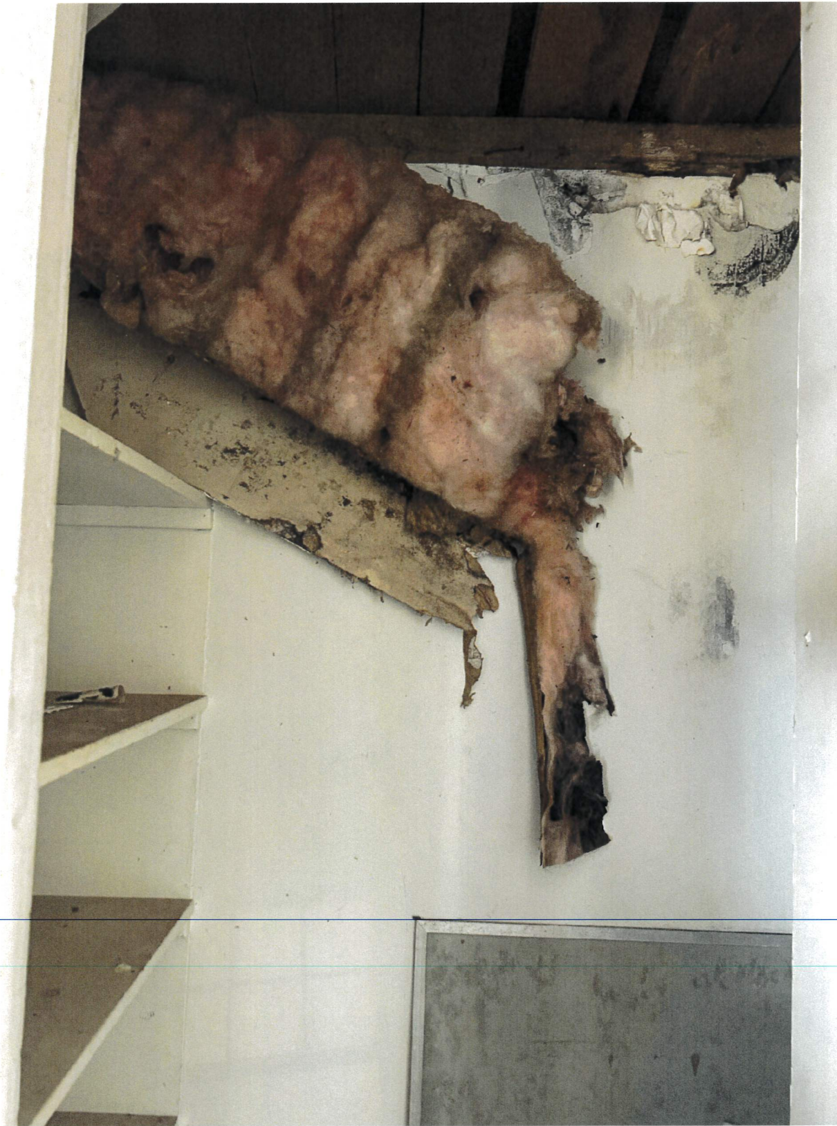
Picture 15: First Floor Closet – Dislodged insulation contaminated with black mold presents severe health hazards and demonstrates prolonged water infiltration and neglect.
