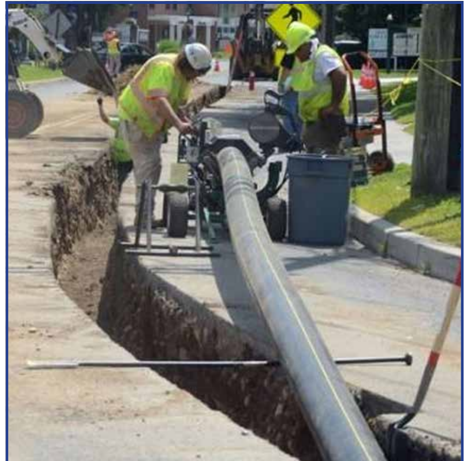
Gas Main Extension in Connecticut
