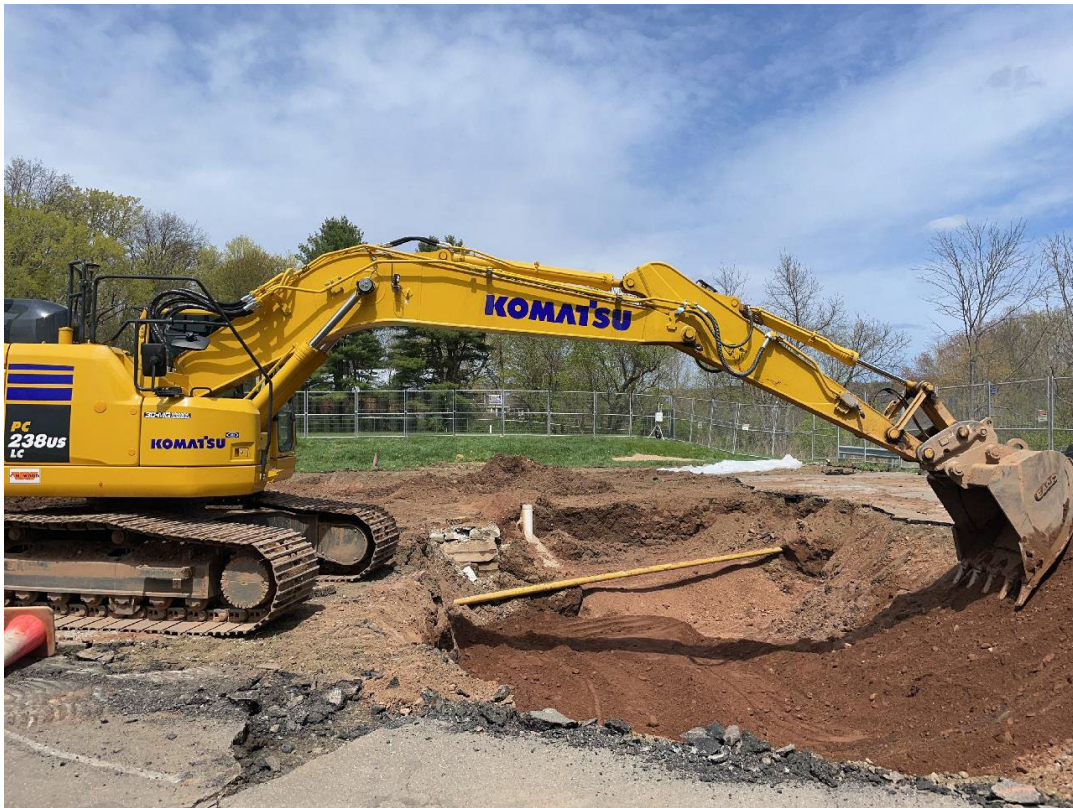
DMC Study Area Phase 2 in progress facing north
