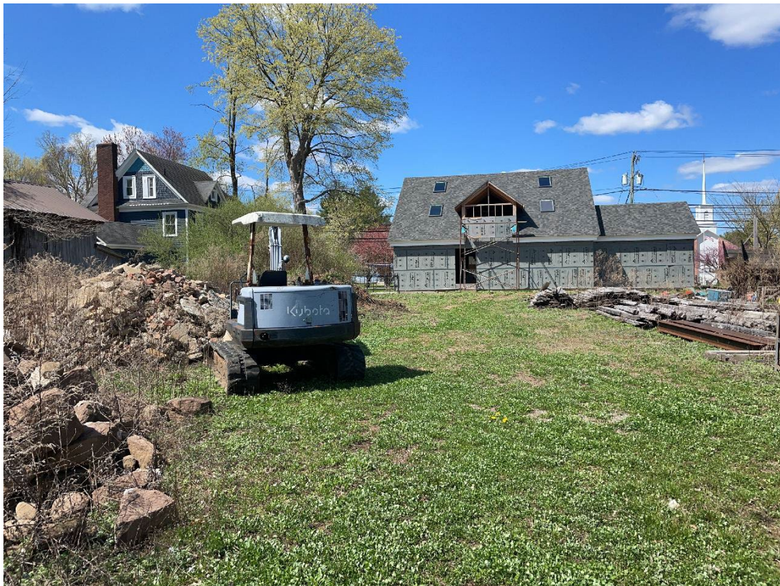
House renovation activities near the MMC Study Area
