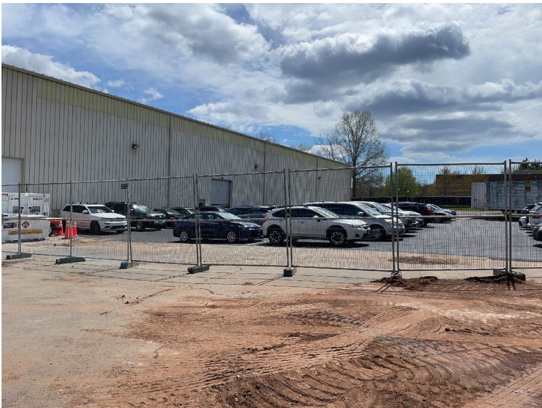
DMC Study Area Phase 1B west of DMC warehouse building
