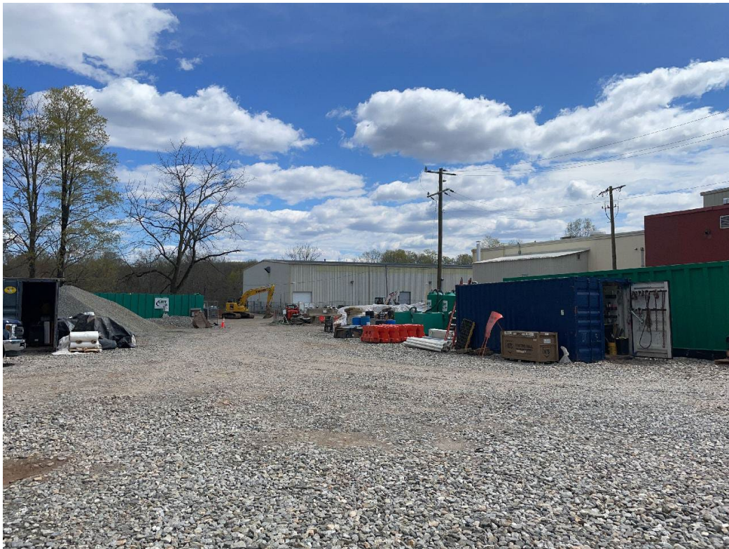
DMC Study Area staging support area and water treatment system
