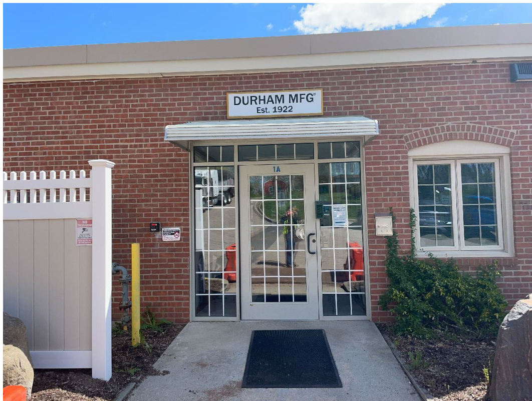
Entrance to main DMC building
