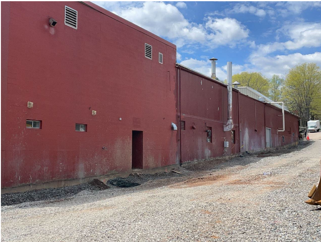
DMC Study Area Phase 1A along north side of DMC building
