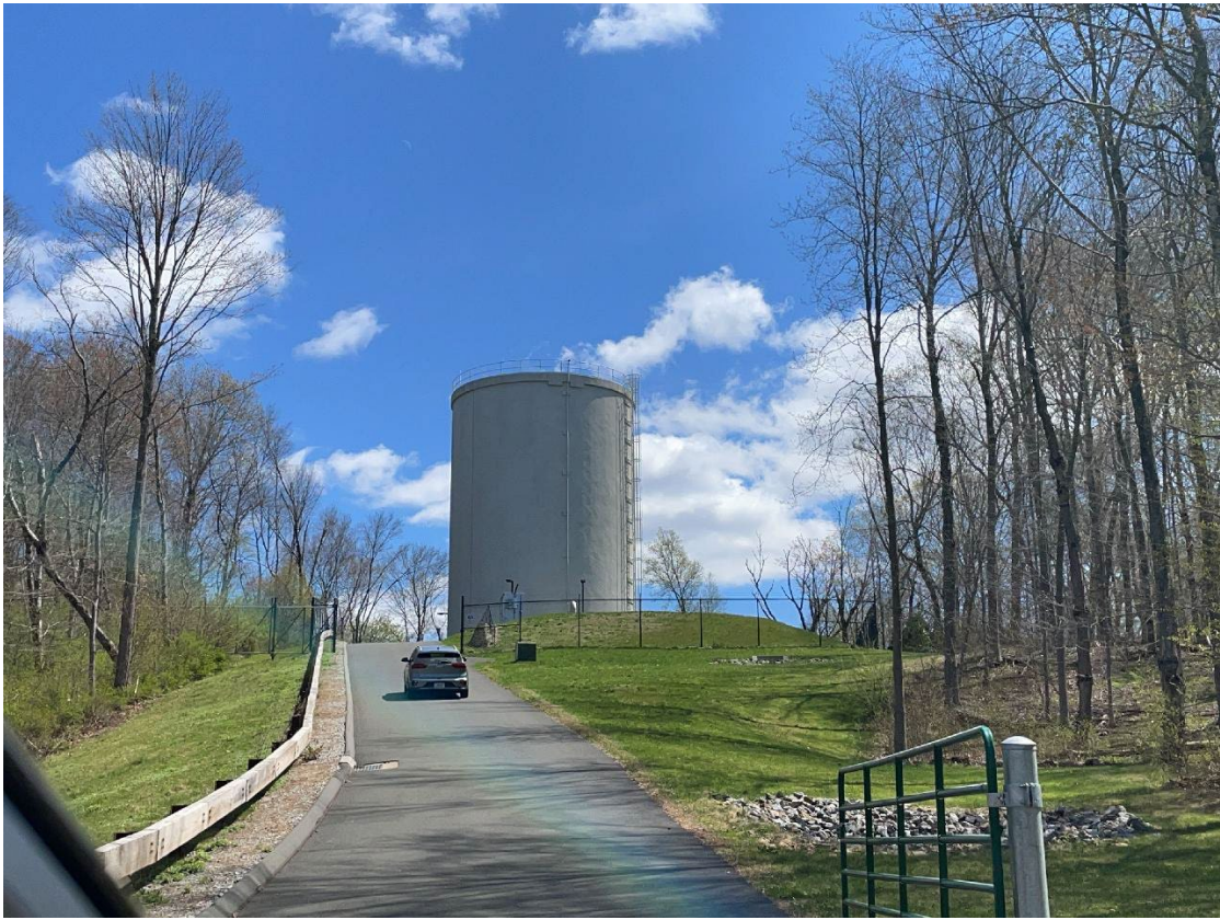
Water tank that services the waterline extension
