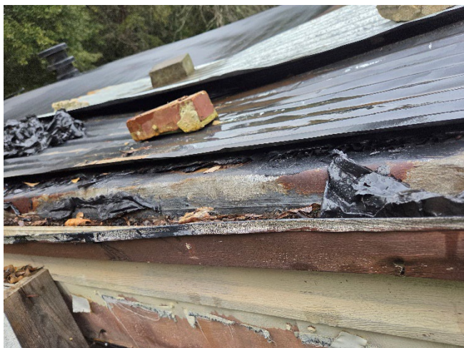
1 Homogeneous Area "A": Roofing paint and flashing
