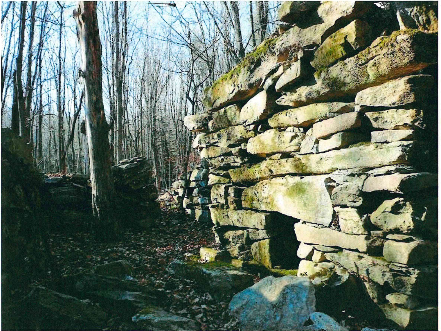
Aquarion Water Company. East Street North (Photo Credit- Henry Moore)
