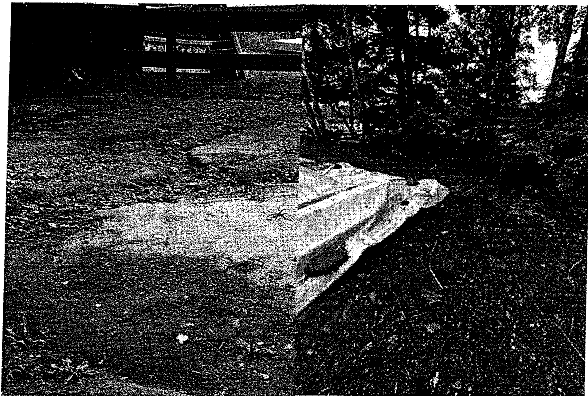
278 West Side Road: Camp Strang (pavilion changed to boat house) Site not stabilized, no E&S controls
