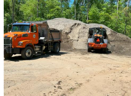
Loading gravel made onsite for use on dirt roads
