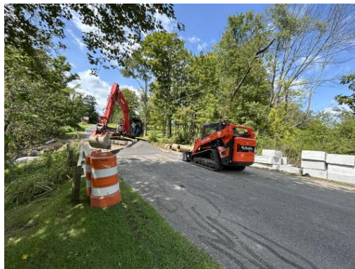
DPW staff working on drainage upgrades on Newcomb Rd.
