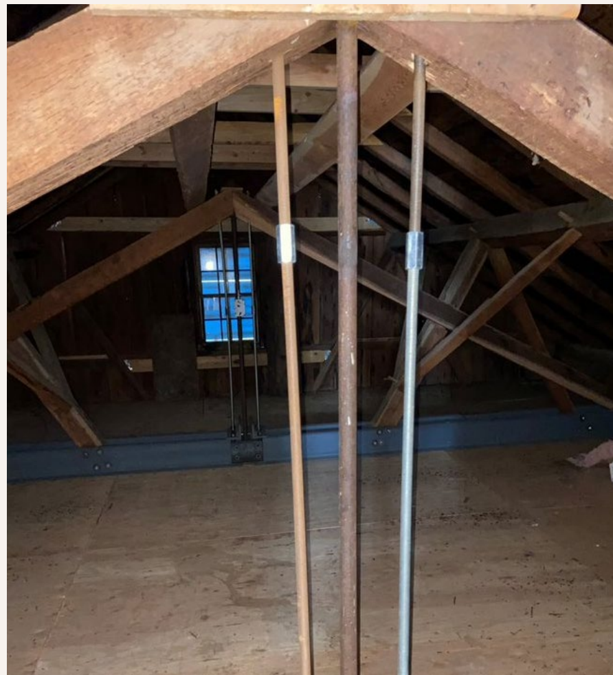
Emergency roof repairs
