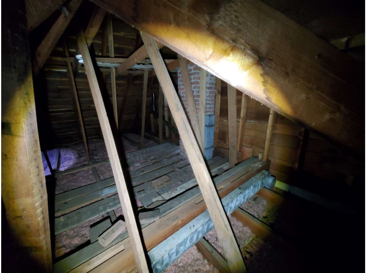
Addendum No. 3 - Photo 3 Upper Attic Looking North 2024-05-01
