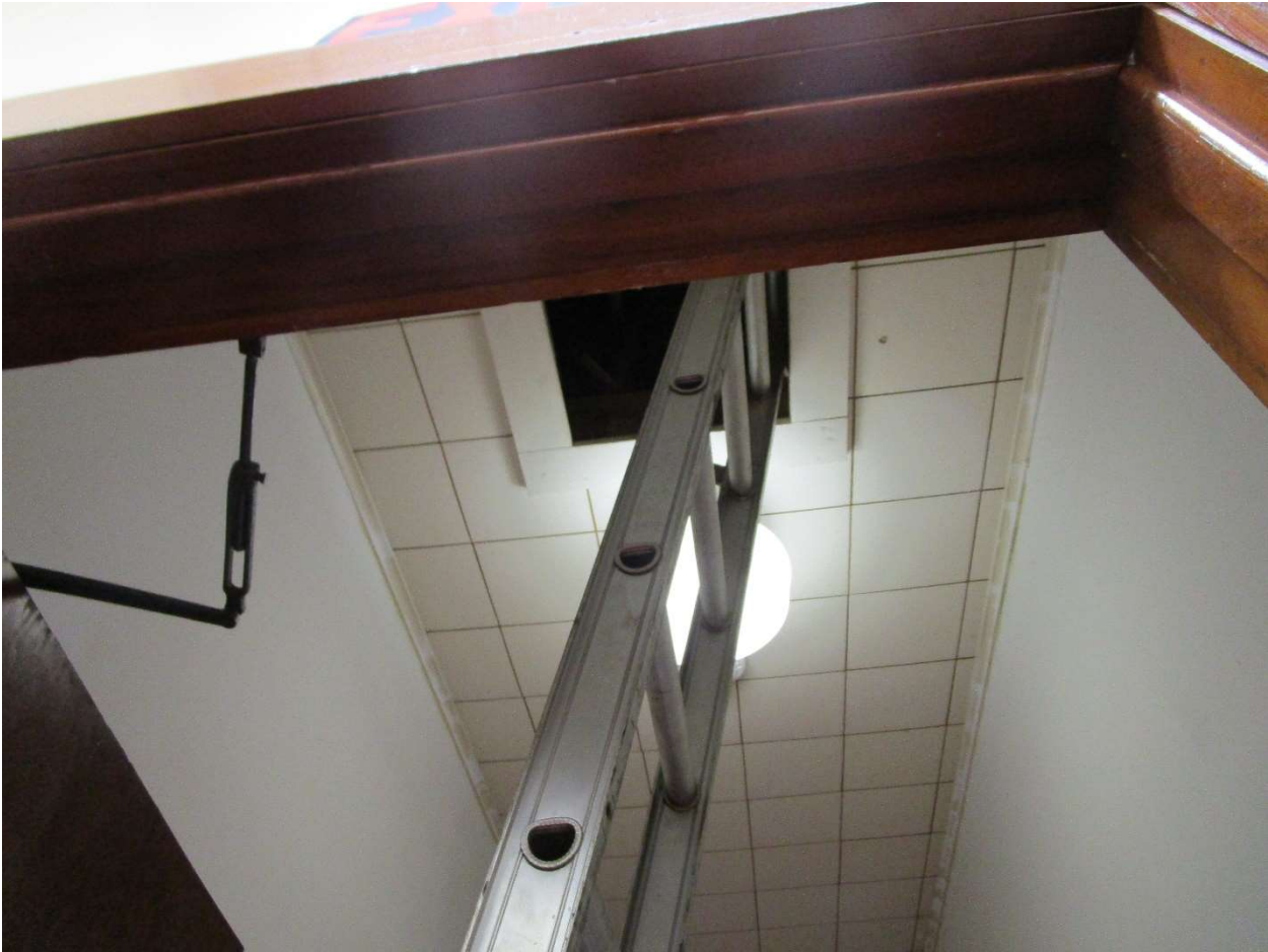
Addendum No. 3 - Photo 5 Second Floor Access to Attic in Stairwell 2024-05-01
