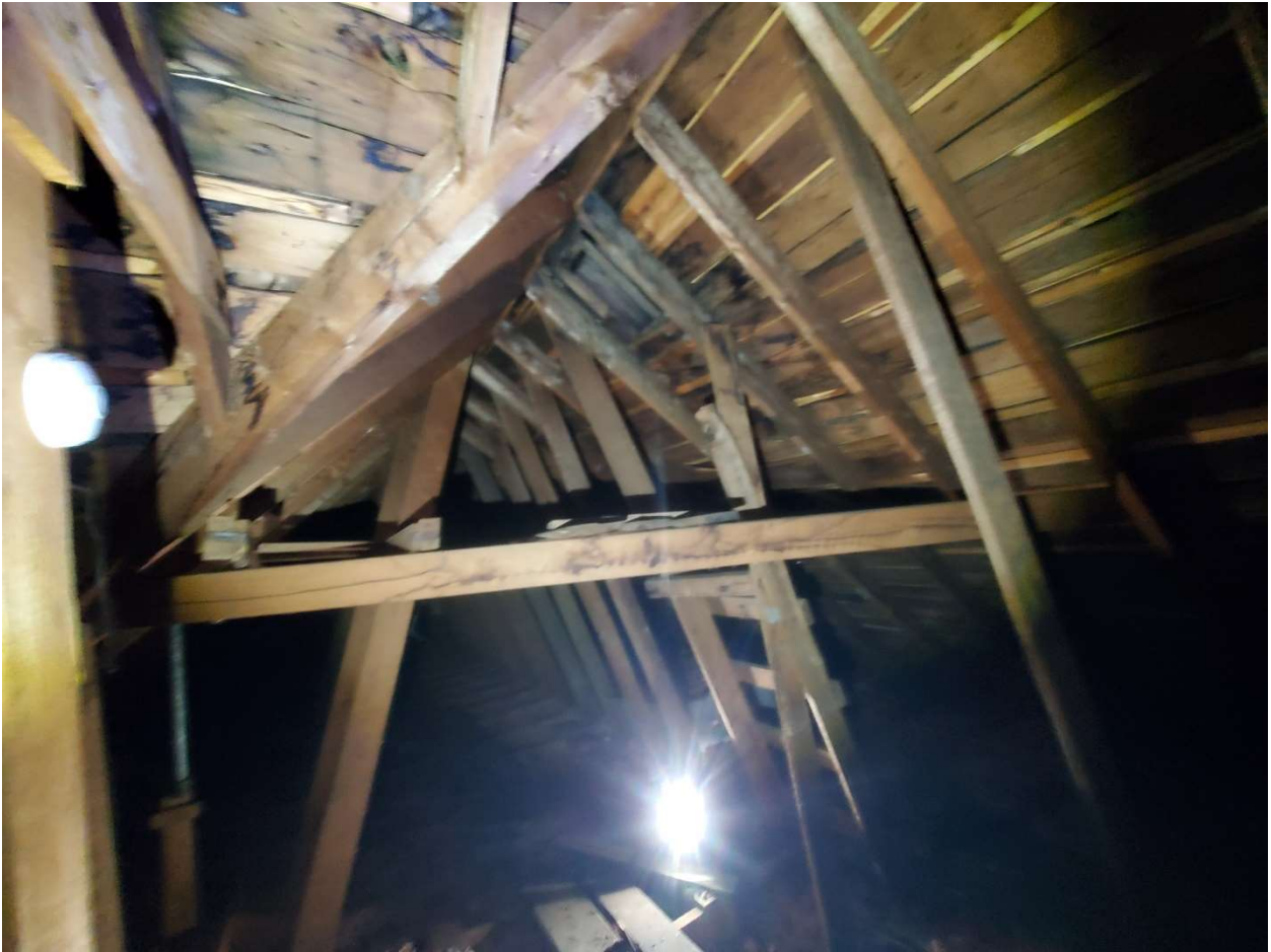
Addendum No. 3 - Photo 4 Upper Attic above the South Wing 2024-05-01
