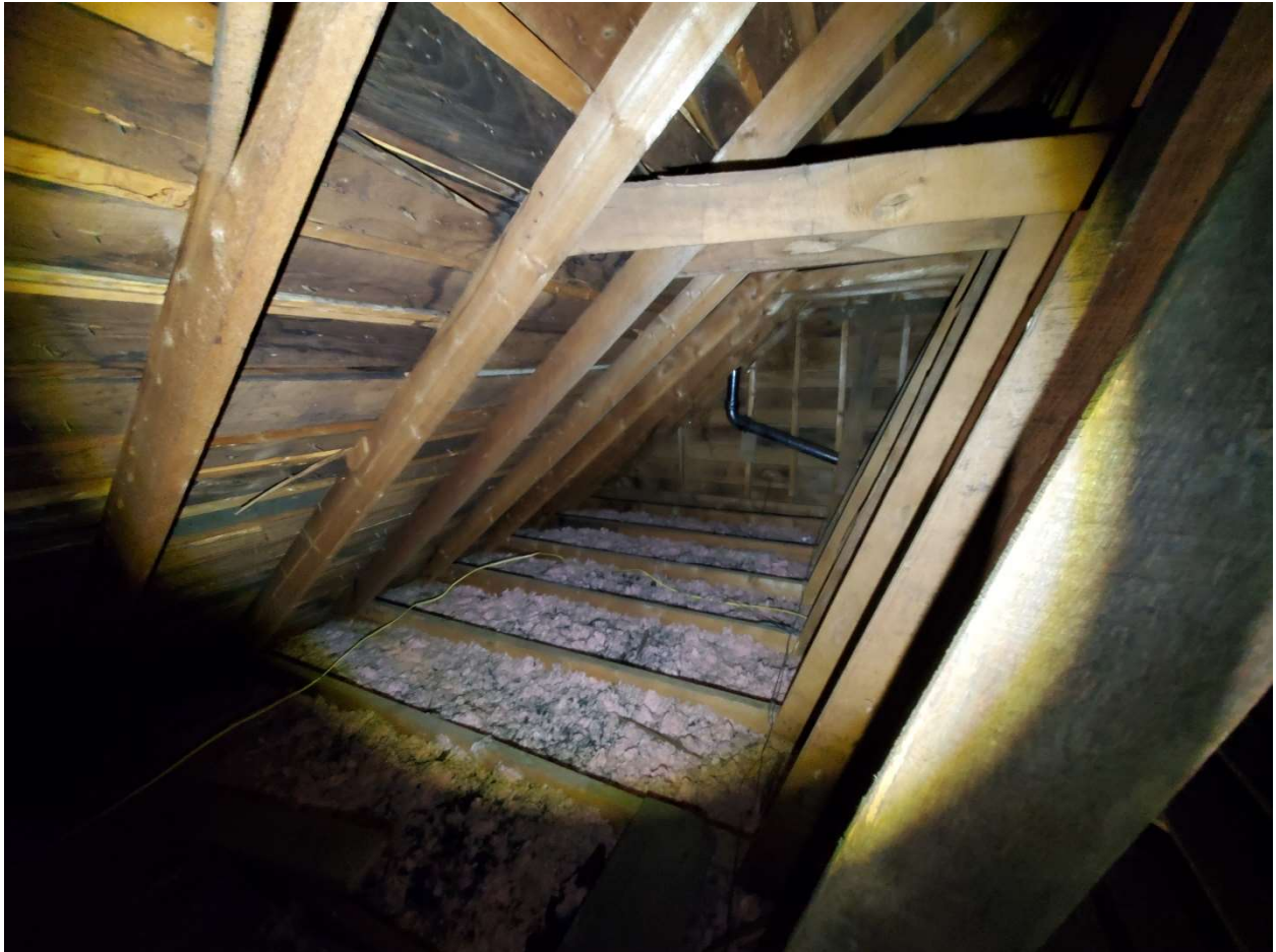
Upper Attic Looking North - 2024-05-01 Plywood sheathing visible above skip sheathing.
