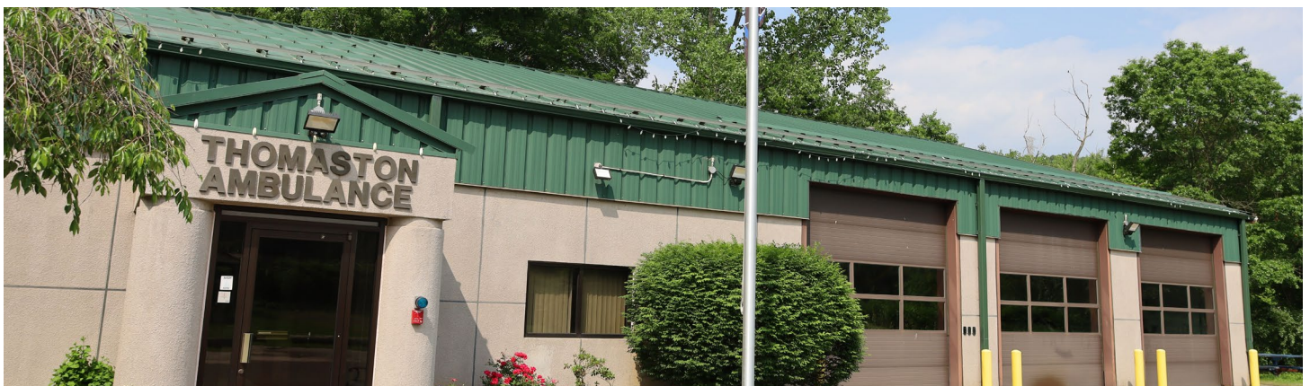
Thomaston Ambulance Headquarters
