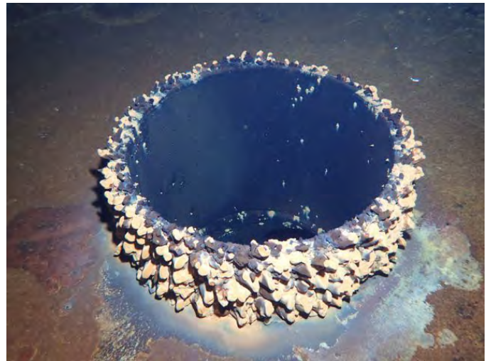
38 16" Inside Diameter Pipe Penetrating The Tank Floor
