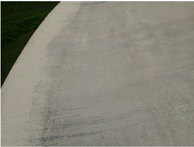
21 Roof Dome With Mild Mildew
