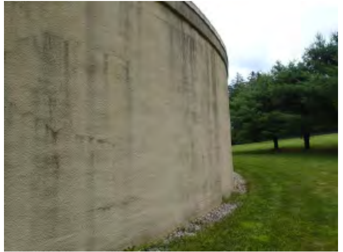
2 Exterior Wall With Coating Loss, Tight Shrinkage Cracks And Mild Mildew
