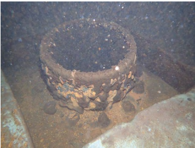
39 16" Inside Diameter Pipe Penetrating The Tank Floor
