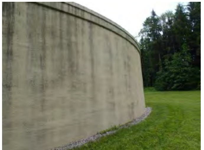
4 Exterior Wall With Coating Loss, Tight Shrinkage Cracks And Mild Mildew
