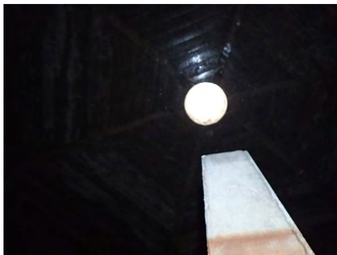
63 Baffle Wall With Heavy Staining
