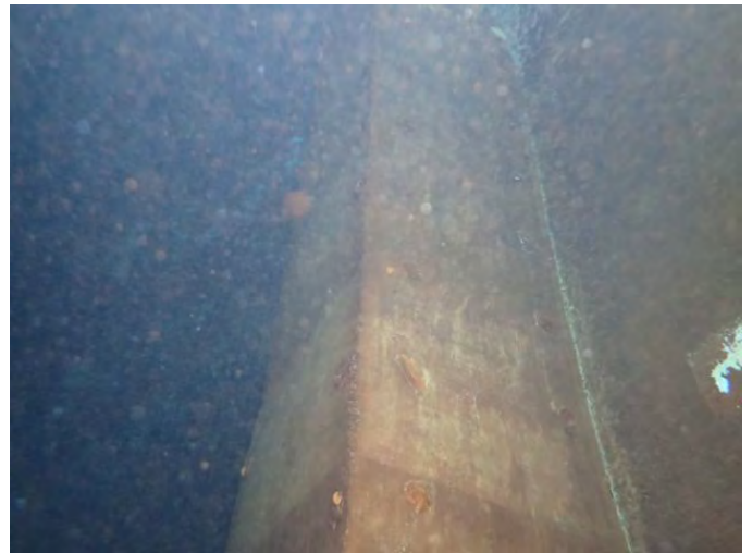
88 Concrete Overflow Box
