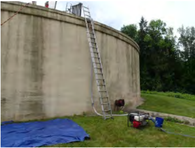
15 Ladder Utilized To Access The Tank Roof
