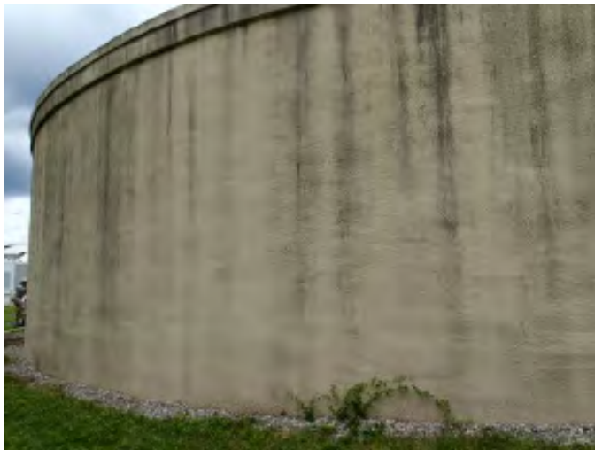
3 Exterior Wall With Coating Loss, Tight Shrinkage Cracks And Mild Mildew
