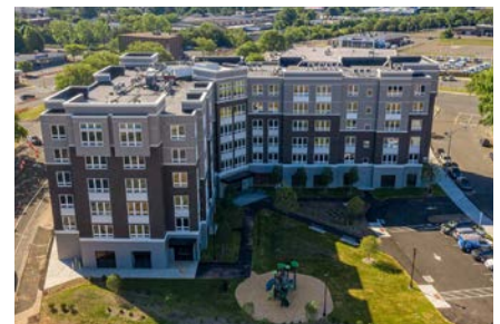
Benesch’s design maximized available space on a tight site to achieve parking, site circulation, and dumpster placement.
