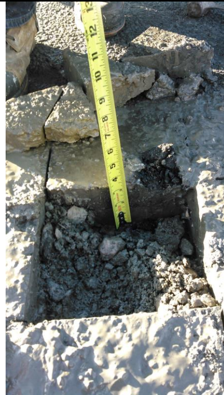
Photo 1. Crumbling Concrete on Deck
