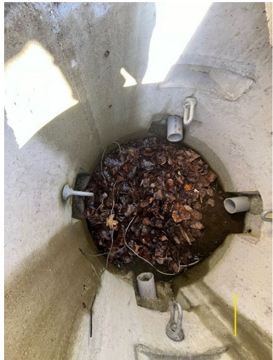
Photo 6: General appearance inside of vaults
