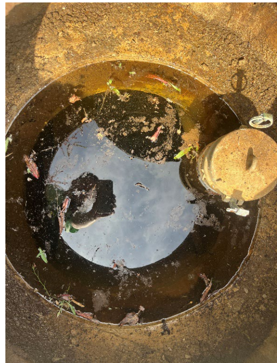
Photo 4: Dust cap intact in SC 2
